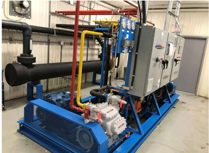
For a single curling rink, it is a good idea to use two or more compressors and two brine pumps. Frequency steered compressors will save energy and will allow for the brine to last longer.
