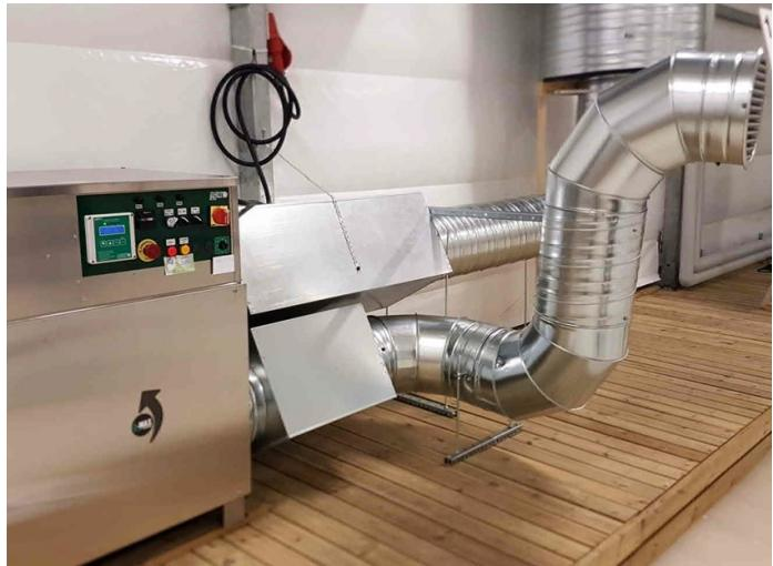
The air in the arena should be heated (see steering and control systems) and controlled by a thermostat. Comfortable and economic air temperature is approximately +7 to +10°C (+44.6 to +50°F) 1.5 m (5 feet) above the ice.
