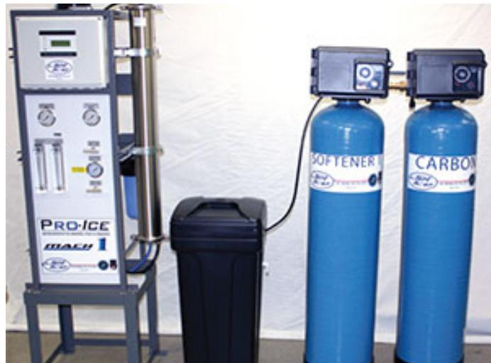
Clean water is a very important requirement in a curling rink. Both to have an energy efficient and hard ice surface and clean water for the pebble. Two purification systems are used in curling rinks, Deionising (DI) or Reversed Osmosis (RO).
