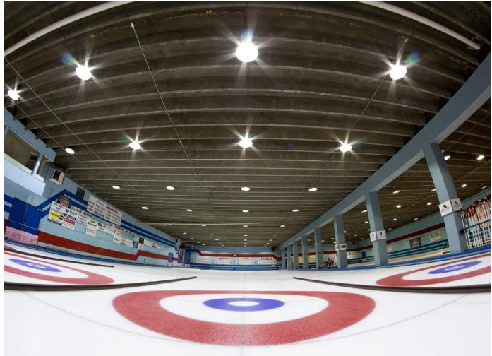
The rink should have good lighting. The lamps should be directed to prevent reflection off the ice that can be distracting for the athletes. A location between the sheets is a good choice but it is recommended to consult with a lighting expert. There should be no heat radiation from the lights.
