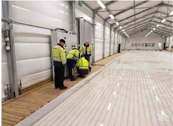
If the curling rink is using the same refrigeration system as a skating rink, the curling rink should have its own brine pumps and its own steering and control system to enable the ice surface temperature to be maintained at the correct stable level.
